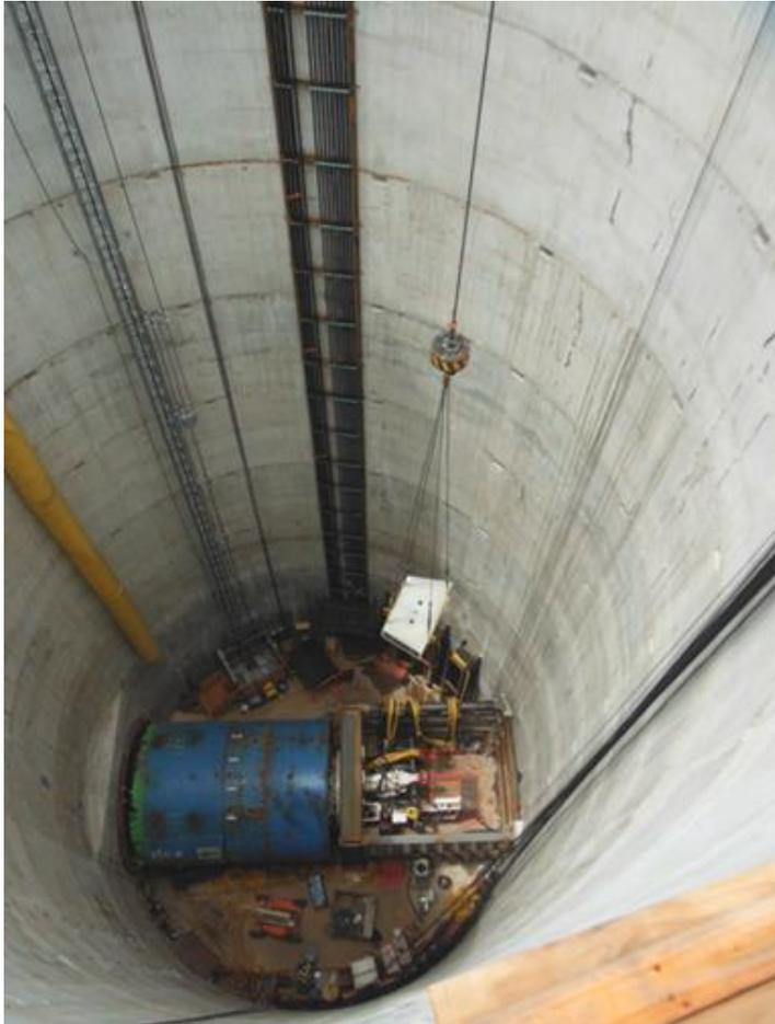
Tunnel Boring Machine in Tunnel at Bottom of Shaft
