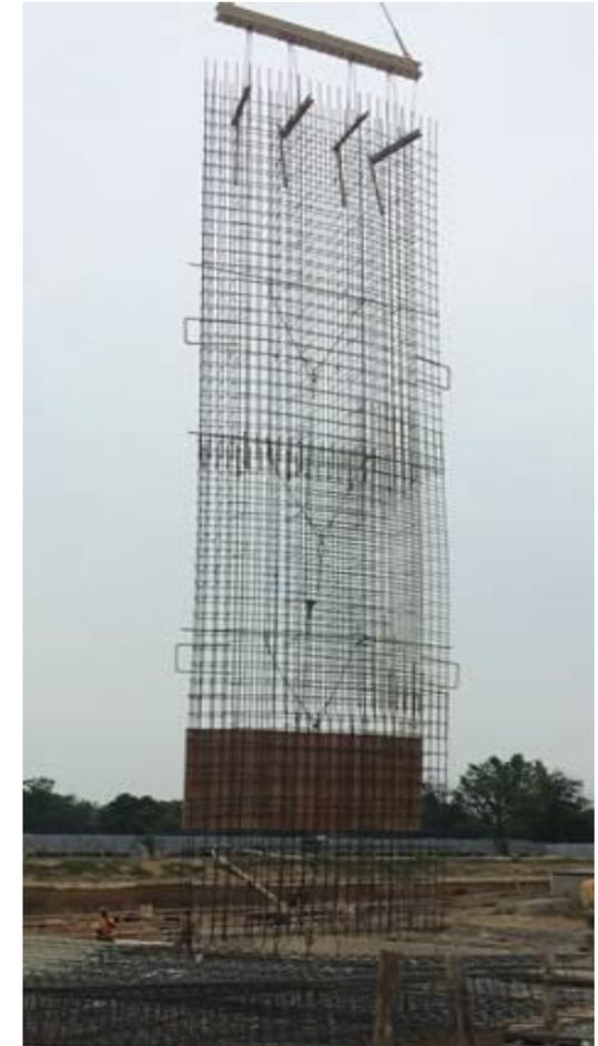
Insert Steel Reinforcing Cage
