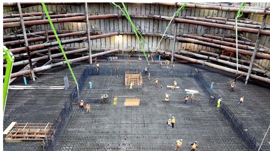
Concrete Placed at Bottom of Excavated Shaft
